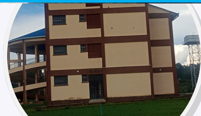
BUILDING AND CIVIL ENGINEERING COMPLEX
